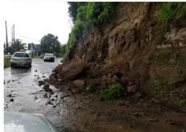
Figure 1: Rockfall in Black Bay
