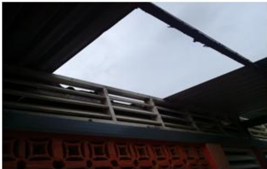
Figure 3: Portion of Roof blown - Soufriere Special Ed. Centre
