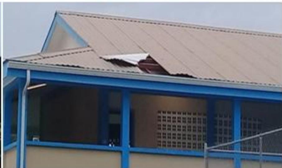
Fig.4: Slight roof damage: Corinth Secondary School
