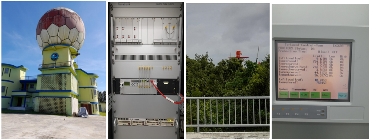
Figure 5. Belize radar components and a sample image of estimated accumulated precipitation
