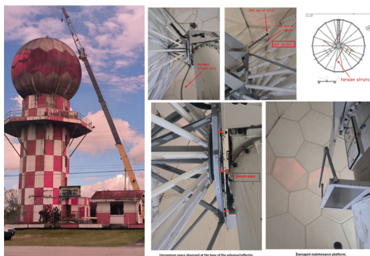
Figure 8. Guyana radar compound and mechanical damage that caused the radar outage
